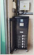
As the store had the capacity to house the power system the team at Energy were able to recommend an EasyGridLite 5000 lithium unit (10.2kWh battery capacity), which has all the same elements as a standard EasyGrid unit but in a lighter housing designed to be kept indoors. The system was expanded to accommodate a larger renewable input of an extended roof mounted 8kW solar– all in providing a robust, sustainable power system for now and moving forward.
