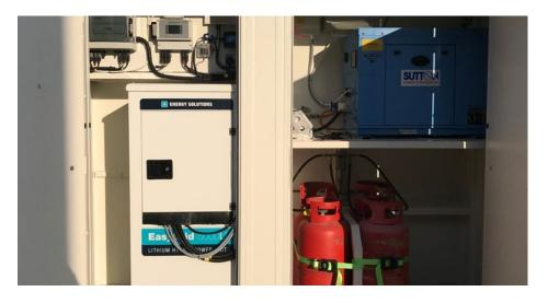
RS French approached Energy Solutions to discuss the power options they could provide and an EasyGrid 5000 Lithium system with solar and wind was specified. The trial container was then built to effectively incorporate the elements of the system, with the solar panels being mounted to the roof and the wind turbine on a pole. Within the container the EasyGrid and generator were housed in their own compartment.
