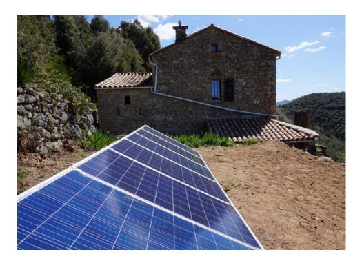
The six solar panels are mounted in a row on a terrace, on the west side of the house, this was done for convenience and proximity to the EasyGrid. The harvested solar power is then transferred to the EasyGrid system set up in a garage below. Electricity is brought into the house via a 30 metre length of armoured cable buried underground and emerging beneath the consumer unit within the house. The JCB G8QX generator is set up in the garage with the EasyGrid.
