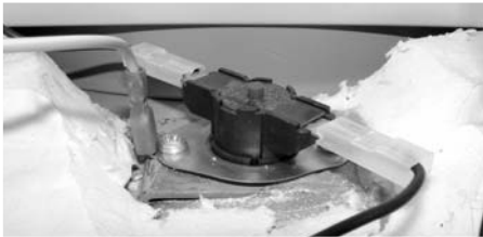
Fig. 26: Safety thermostat reset button.
